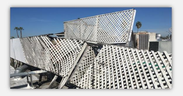
Though these lattice panels provide up to 50% opening, they still failed under 60 MPH winds.
