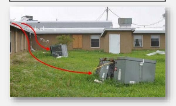
During high winds this mechanical equipment was removed from its foundations and the roof itself. Even mechanical equipment on a low roof is susceptible to high winds without an enclosure.
