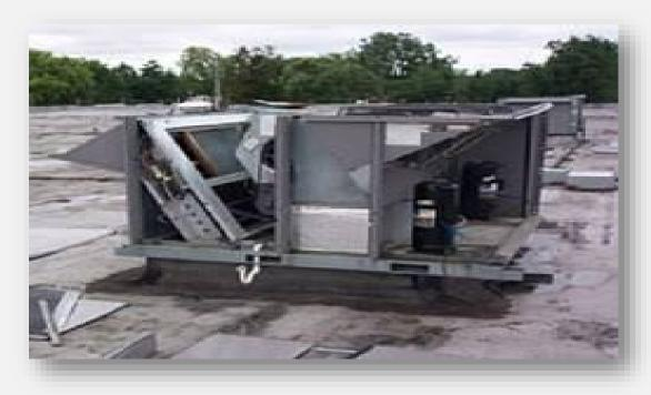
This mechanical equipment was screened, however, during high winds the screening was compromised and caused damage to the equipment.
