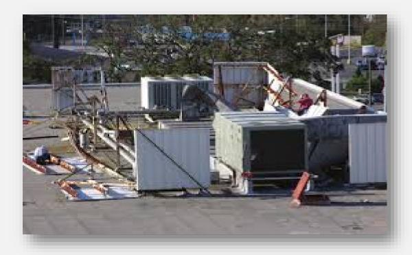
High winds resulted in damage to this mechanical equipment. The equipment was screened by a non-engineered enclosure that was wood framed and corrugated steel application.
