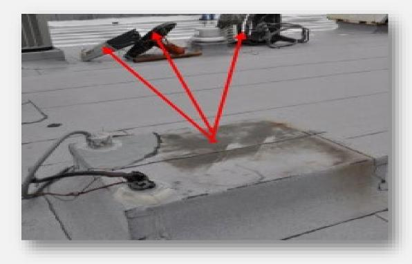
This mechanical equipment and associated screening was detached from the top of a building as a result of high winds.
